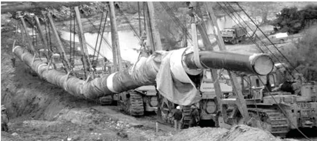
Figure (11) Pipeline construction
